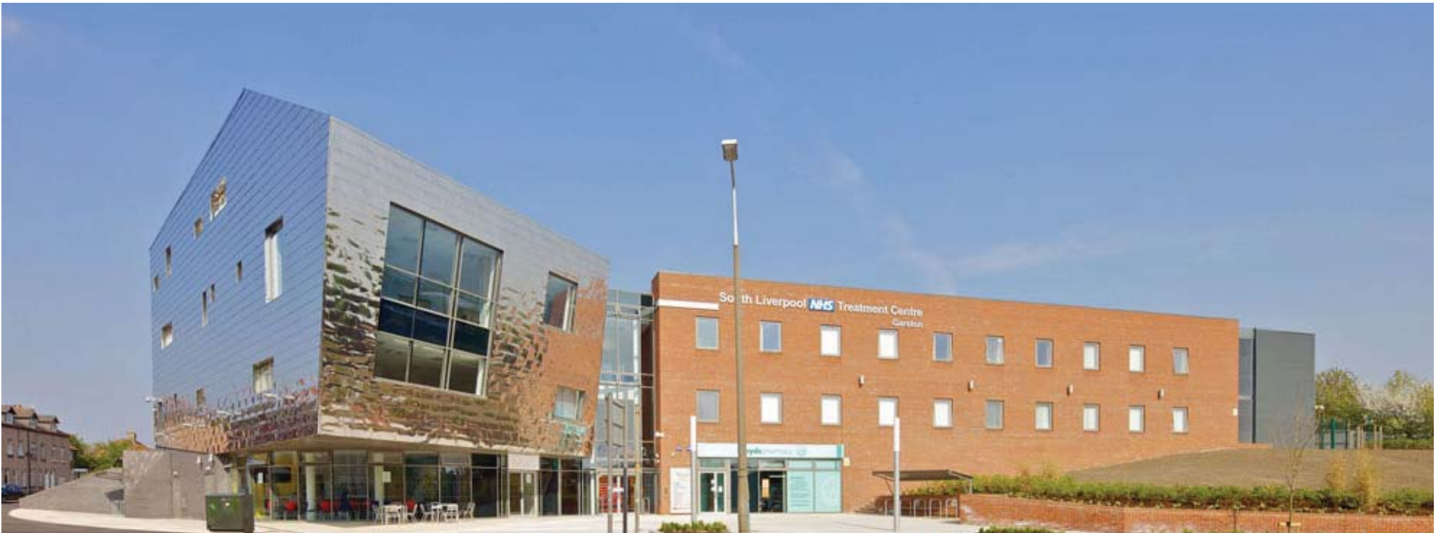
Stainless steel clad 'zig-zag' cantilevers over the Main Entrance
